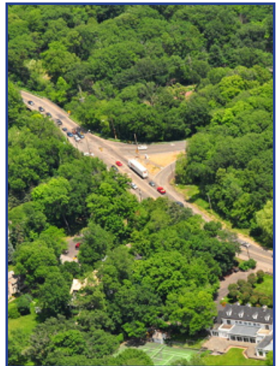
McGinty/Eastman Lane/Bushaway Road Intersection from South
